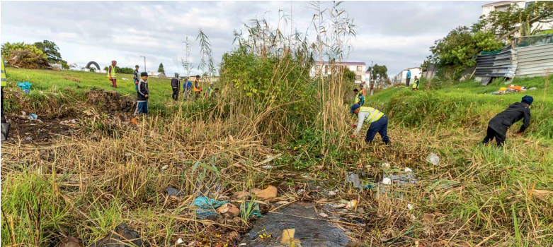
Many hands, light work: As part of its winter preparedness programme, the City cleared the Macassar canal of excess debris, vegetation and silt that may restrict the flow of water once the winter rains come. The labour-intensive work was carried out by a large team.
