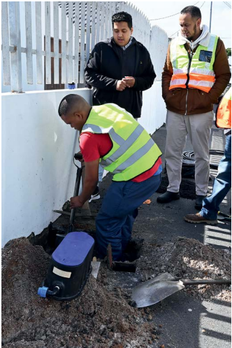
Getting stuck in: Mayoral Committee member for Water and Sanitation Cllr Zahid Badroodien (in the black jacket) with a team on-site in Athlone carrying out a water meter replacement.
